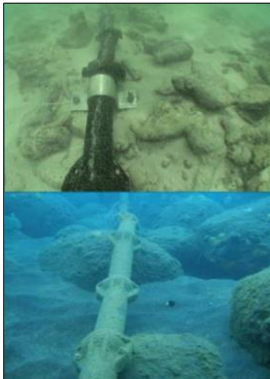
Figure 24: Articulation on submarine cables. Pinning on hard substrate is shown
