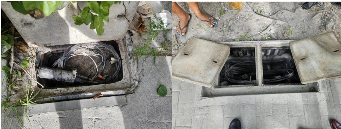
Figure 28: Example of manholes filled with sand (left) and relatively clean (right)
