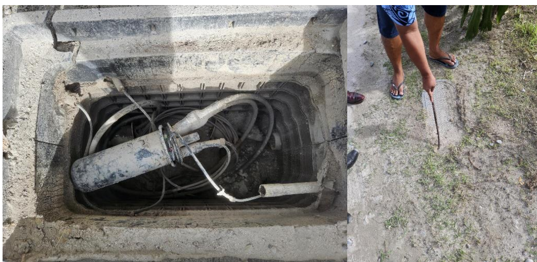
Figure 29: Examples of smaller pit with drops (small conduits) directly to the homes
