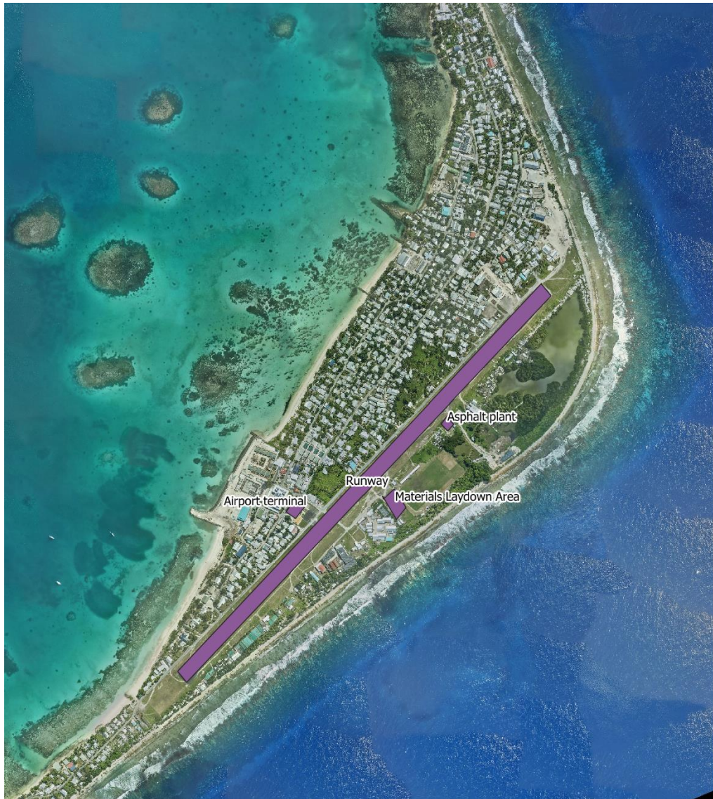
Figure 1: shows all project site for the TuSRAP including Airport terminal, runway, asphalt plant and lay down area for project materials.
