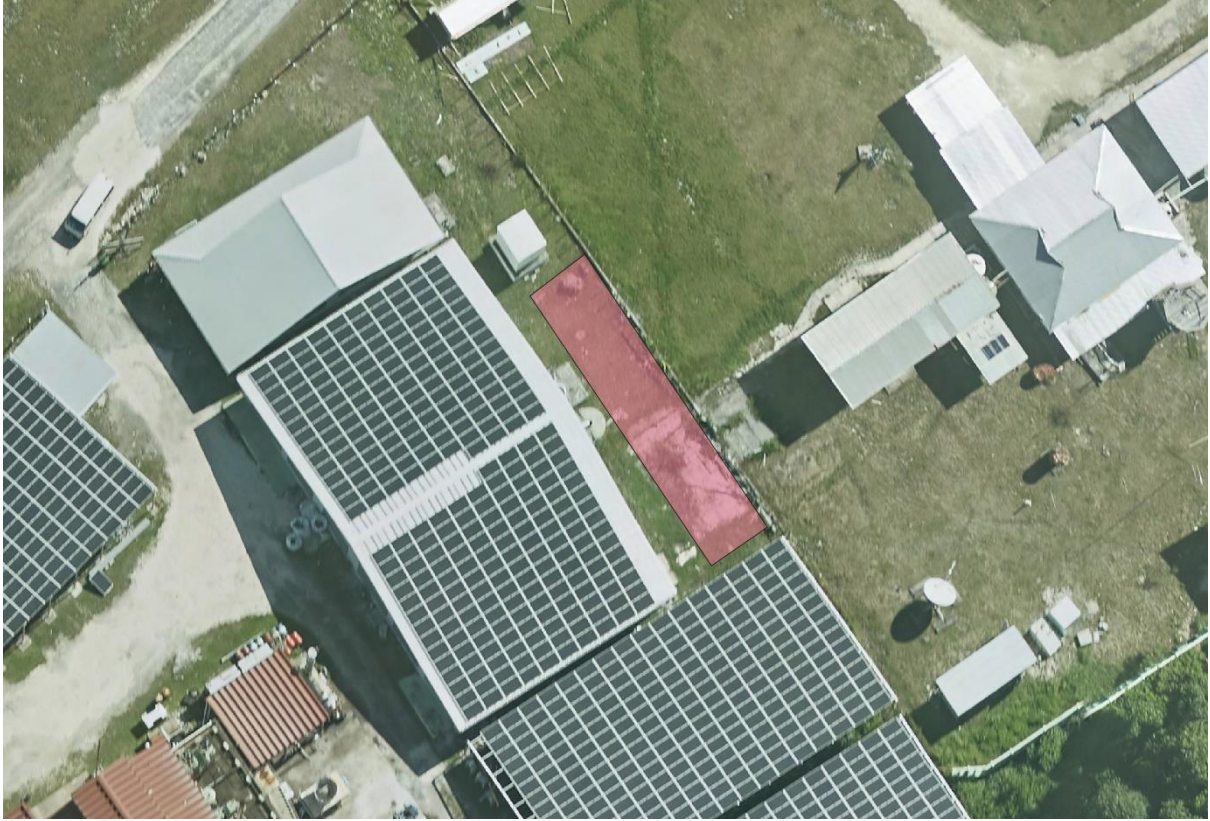
Figure 8: The location site of solar battery (pink colour) within the TEC compound.
