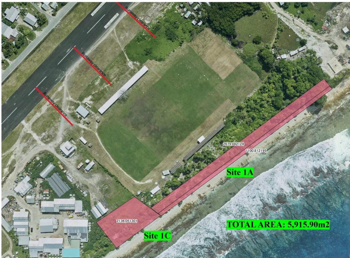
Figure 1: The two sites for the project (Site 1A, ,1C) identified for installing solar PV arrays.
